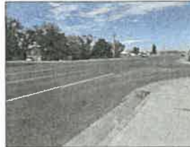
4000 SOUTH LOOKING WEST
