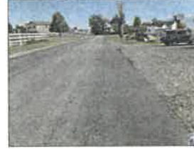
NORTH LEG OF 4300 WEST LOOKING NORTH
