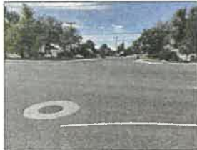
SOUTH LEG OF 4300 WEST LOOKING SOUTH
