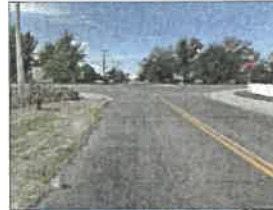
NORTH LEG OF 4300 WEST LOOKING SOUTH
